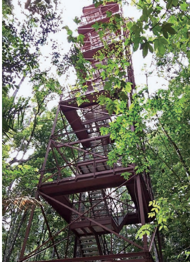
Tower for observation of forest canopy (ZF-2 Tower: 40m+10m)
